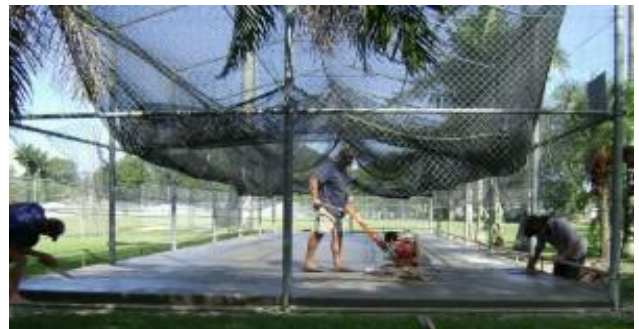
Rick Robinson puts the final touches to the slab.
