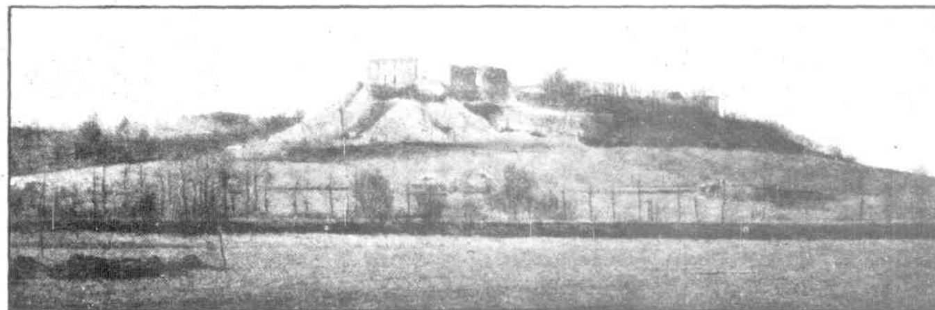
AFTER IT WAS BLOWN UP BY 25 TONS OF GERMAN EXPLOSIVE.
